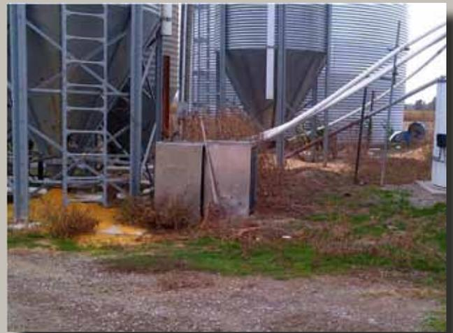
Feed spills and leaks can lead to inaccurate weights on weigh cells, attract rodents and hurt feed efficiency yearly calculations.
